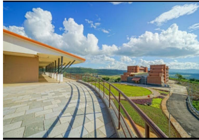
Terrace and residential block
